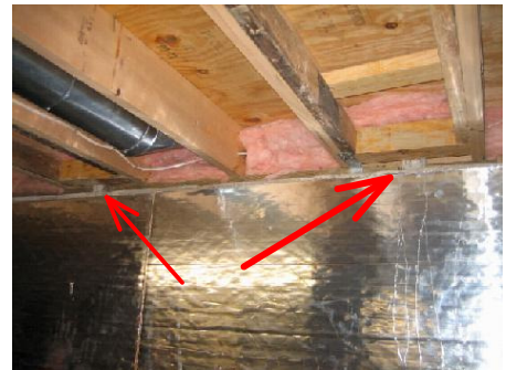
unable to determine bracing need, please contact a qualified structural eng to evaluate.
