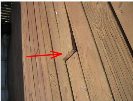
loose boards need to be properly secured.
