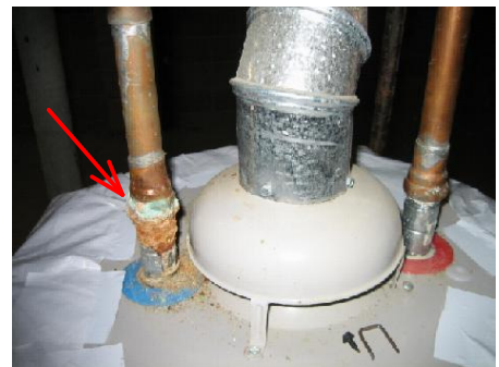
excessive rust at cold union on water heater
