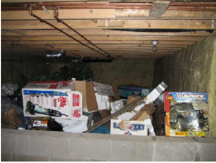
crawl space access
