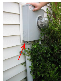
earth settle has pulled protective conduit from service meter.
