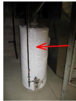
protective cover on water heater does not allow access to heater information.
