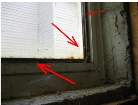
cracked or missing glass
