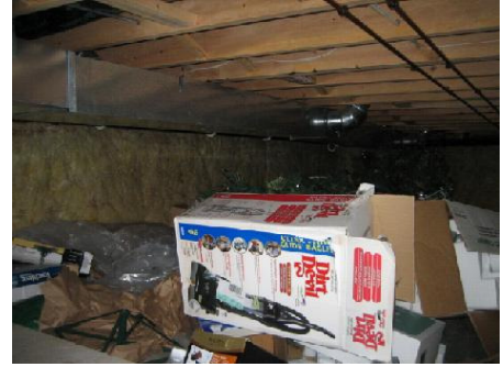
crawl space access
