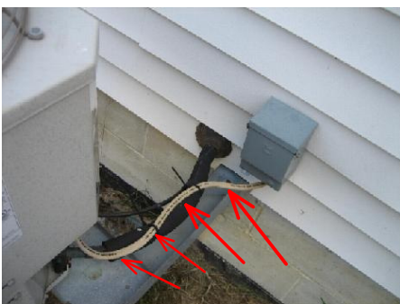
uncommon method for exterior wire
