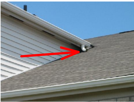
drain should be extended to gutter below
