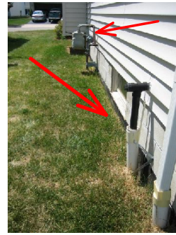
negative slope (swale) : excessive rust on gas pipe
