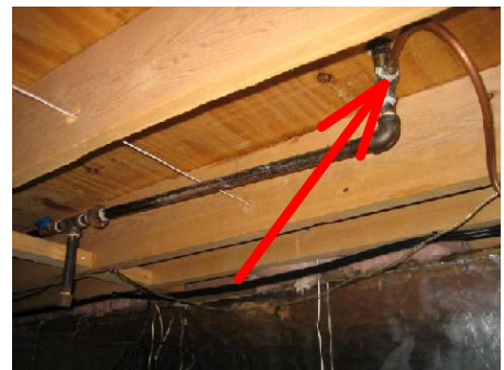
gas leak to fireplace
