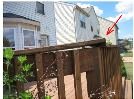
loose boards need to be properly secured.
